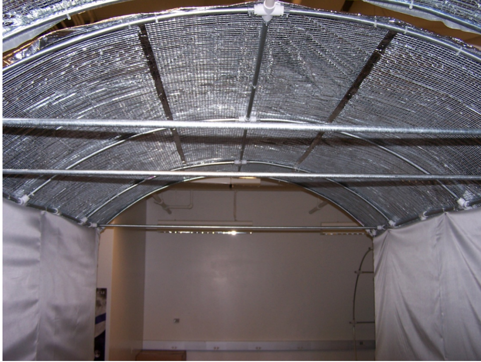
Figure 25: Upper section of LSAM Prototype with electrical conduit as structure.
